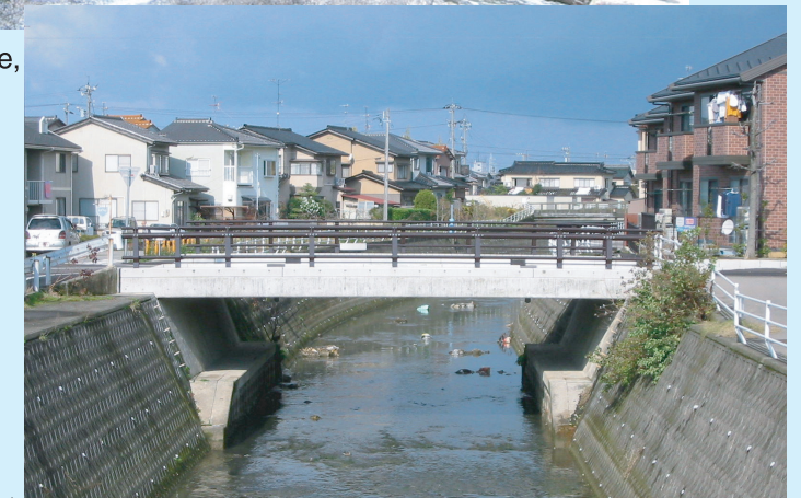
Works for changing the superstructure of Tarota Bridge, Bridge length: 13.10m Kanazawa City, Ishikawa Pref. (Built in September, 2004)
